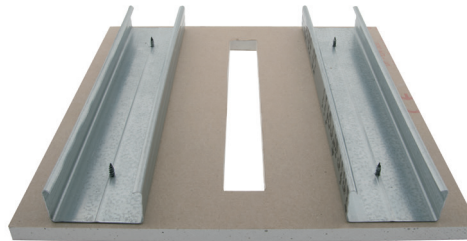
2. Cutting out the plasterboard
